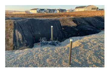
Deep pipes installed with pressure test on all pipes
