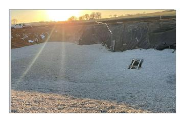
Deep pool main drain piping completed, fabric laid and 12" clear stone installed
